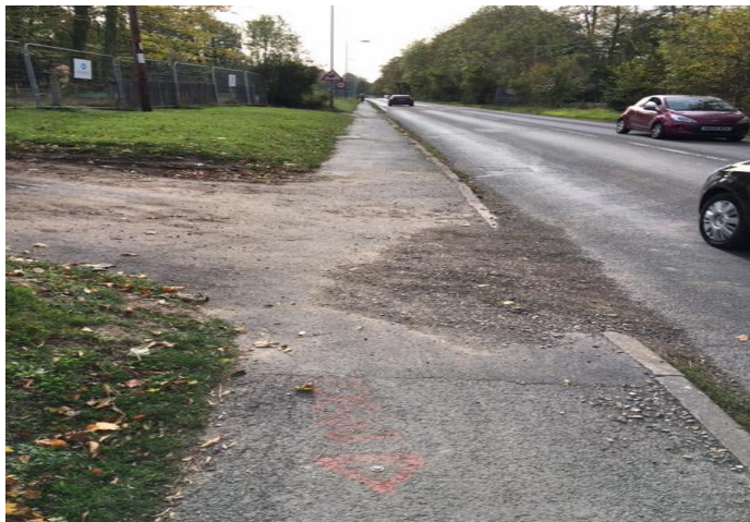
Looking along the A338 by the Early Years Centre
